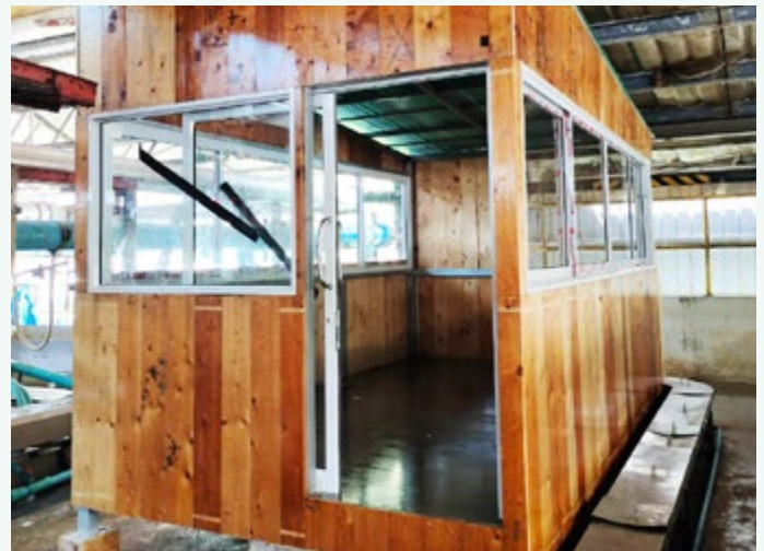
"upcycled disused machine boxes to a mini office in the production line"
